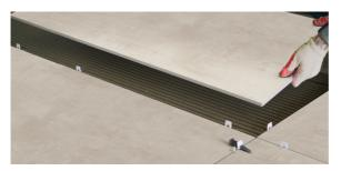
16. Especially when laying rectangular and large size products such as 30x120 and 60x120 cm. the Ceramic Leveling System (wedge joint application) consisting of wedges, holders and forceps should be used to adhere them at regular joint intervals and at an even level. As in the example, using wedge wedges close to the corners and increasing the number in the middle as the tile size grows will make the application much smoother.
