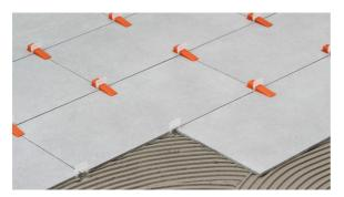
17. For products with an aspect ratio of more than 2 times such as 30x120 (120/30 = 4), as we have stated in the product boxes, the applications should be made in a 1/3 ratio. Information on the box is as follows. This means that for a product with a long side of 120 cm, it is tiled with a shift of 120 cm x (1/3) = 40 cm.
